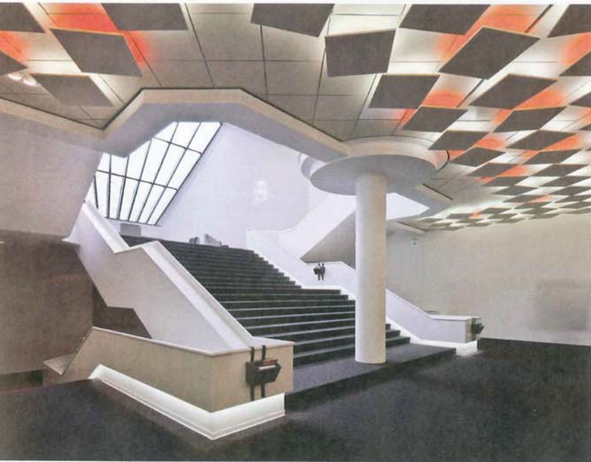
Below: The felt-clad acoustic tiles conceal lights that not only change color and intensity but act as way-finding devices and cues for audience members to take their seats.
