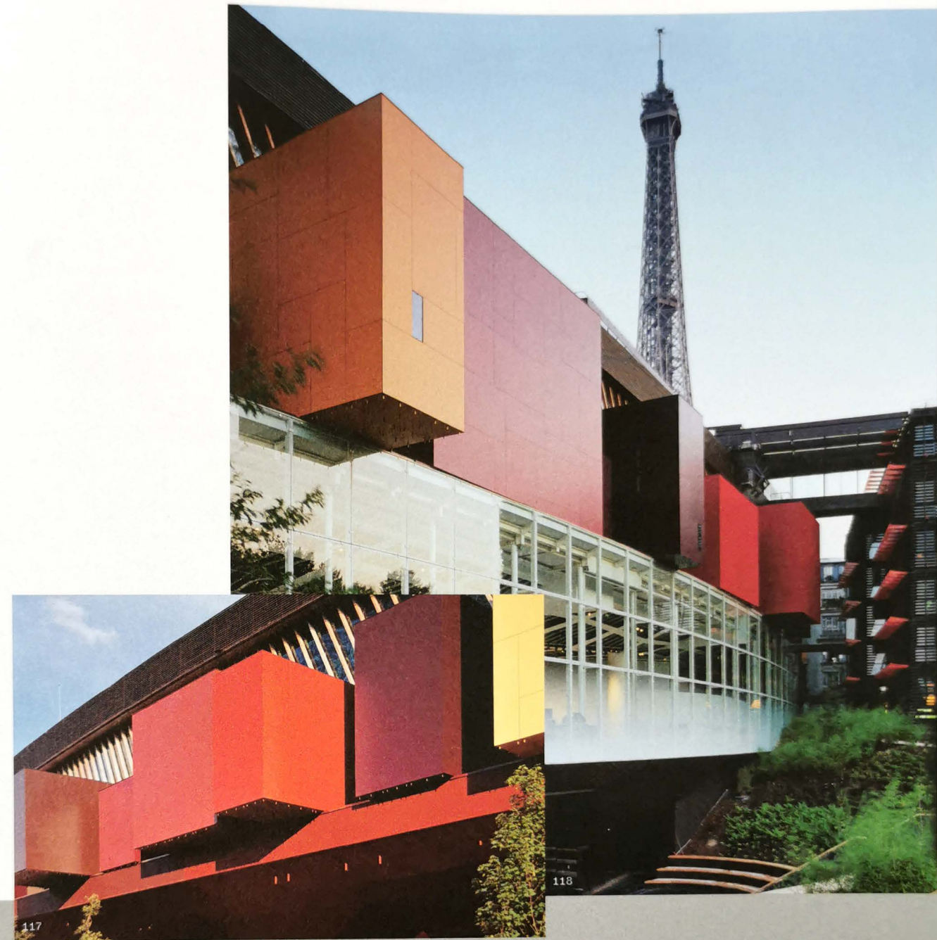
Musée Du Quai Branly (Paris, France) by Ateliers Jean Nouvel. Made with Trespa Meteon.
